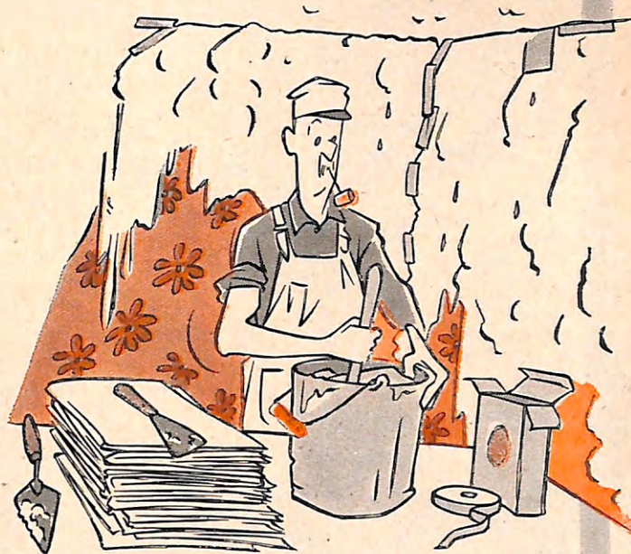
Caulk a third floor room with a mash made of newspapers soaked in washing soda.
