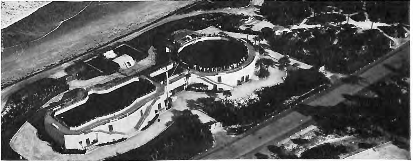
An airplane view of Marineland, showing the two large tanks and the connecting flume.
