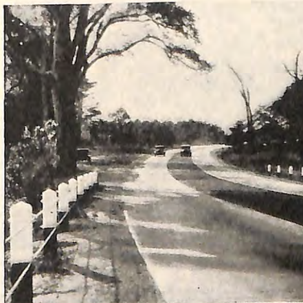
The rough macadam center lane prompts drivers to keep to the right.
