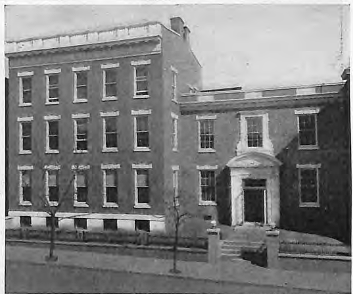
The new Home of Lancaster, Pa., Lodge, a structure remodeled a short time ago at a cost of $50,000; and since formally dedicated
