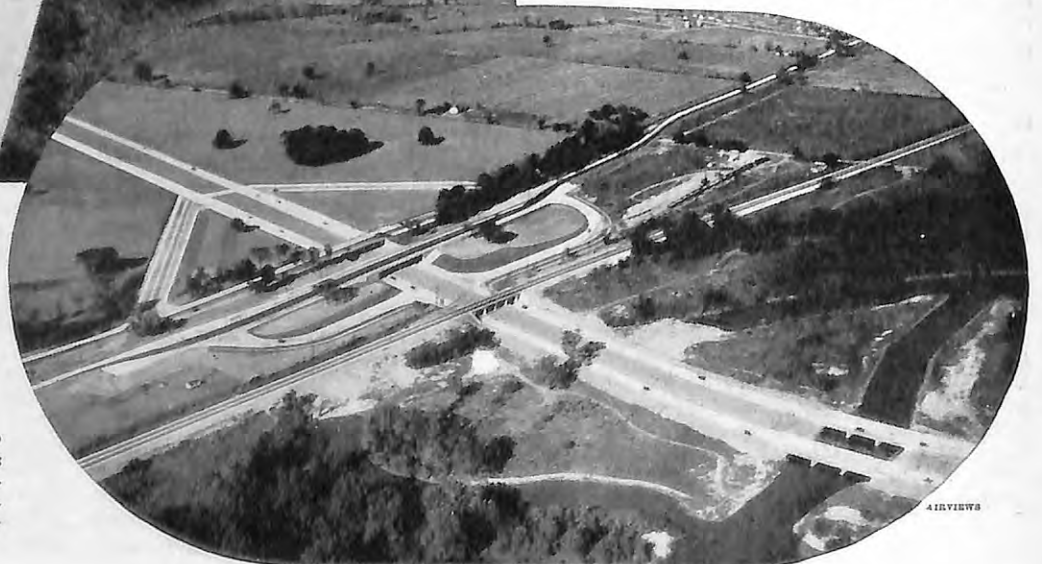
This grade separation of two Michigan super-highways involves two bridges crossing two highways, a railroad and the Rouge River
