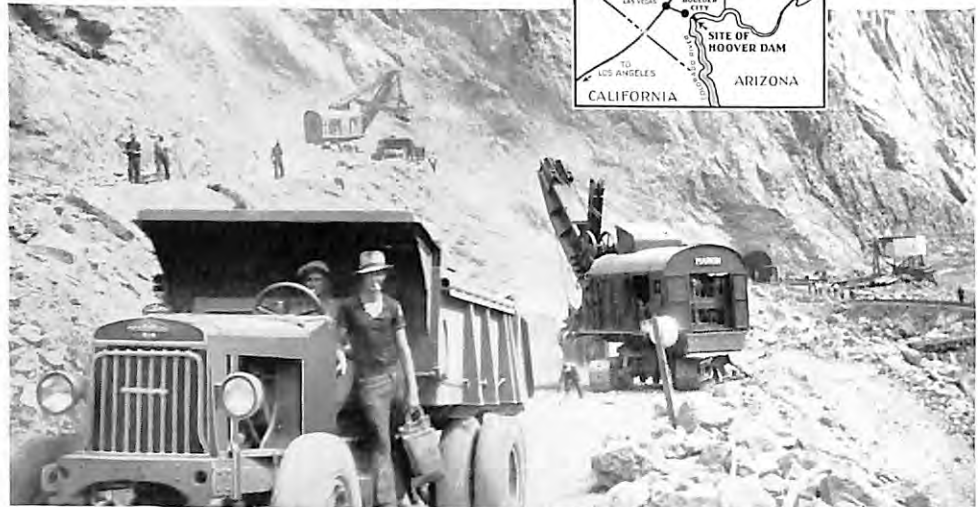
One of the International heavy-duty trucks working at Hoover Dam. The open hood is expressive of the intense heat in the canyon, rising as high as 128 degrees. The boulder-proof armored cab is further evidence of conditions encountered. Note, at right of shovel, the entrance to an auxiliary tunnel used in construction of the great diversion tunnels that will extend three miles through solid rock.
