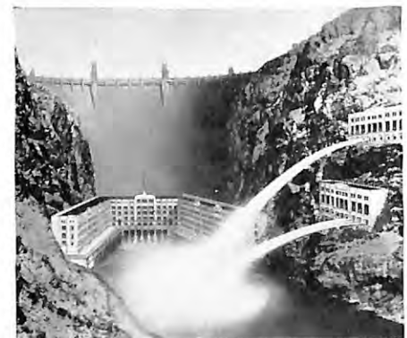
Hoover Dam as it will look on completion, towering 730 feet above foundation rock, with power houses on both banks of the river. The dam will be nearly 1200 feet long, 45 feet thick at the top, and 650 feet thick at the base. This barrier will form a reservoir 115 miles in length with a shore line of 550 miles and an area of 227 square miles, the largest artificial lake in the world.
