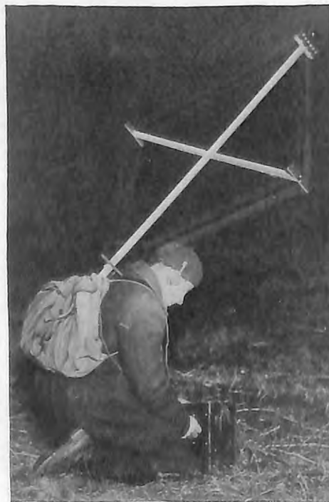
Trying to locate the rocket by catching, on a swinging receiver, the automatic buzzing signals which are sent by its short wave sender
