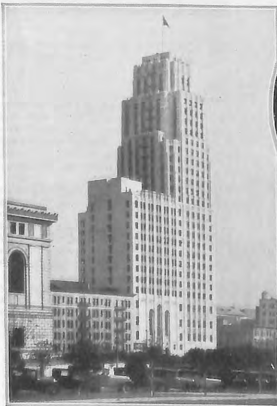
In a building with a splendid design for vertical emphasis and for outline against the sky, the twenty-eight story San Francisco structure pictured above combines a hotel and the Temple of the M. E. Church
