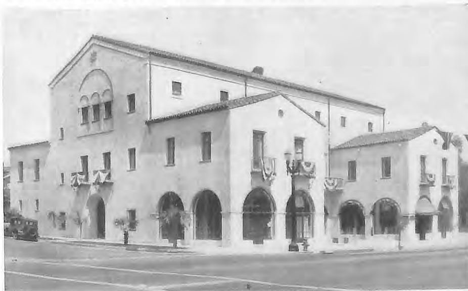
The splendid new Home of Alhambra, Calif., Lodge, No. 1328, recently dedicated
