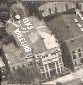
View of aerial marker on roof of Wheeling, W. Va., B. P. O. Elks Lodge, No. 28
