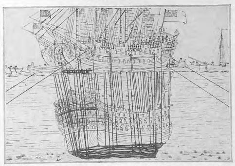
Two old drawings showing the early application of methods still used to raise wrecks. At left, compressed air is being pumped in. Above, a hulk is being floated to shallow water
