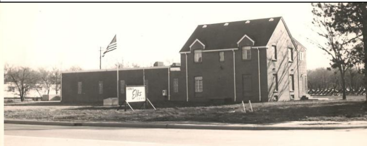
The "old house" after the first phase of the building expansion project.
